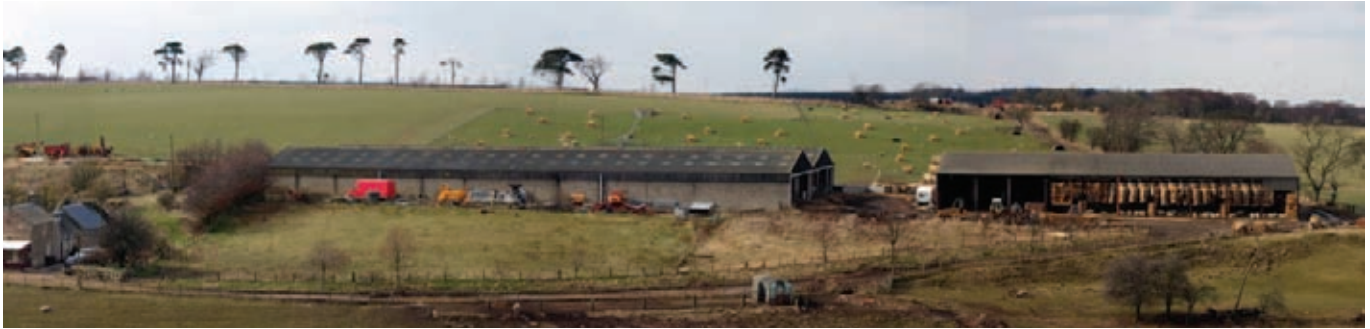
Viewpoint 1, showing the farm buildings with lambing fields in the background, and young planting already established along the ridgeline to replace the pine shelterbelt
